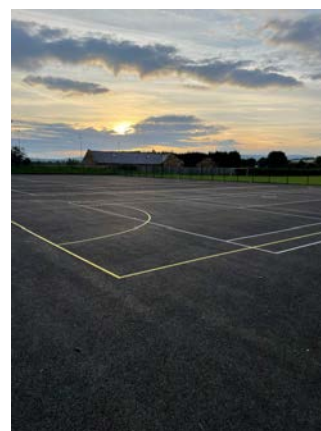
The newly resurfaced courts
