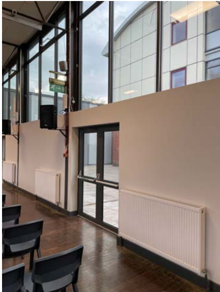
New fire doors and windows in the hall
